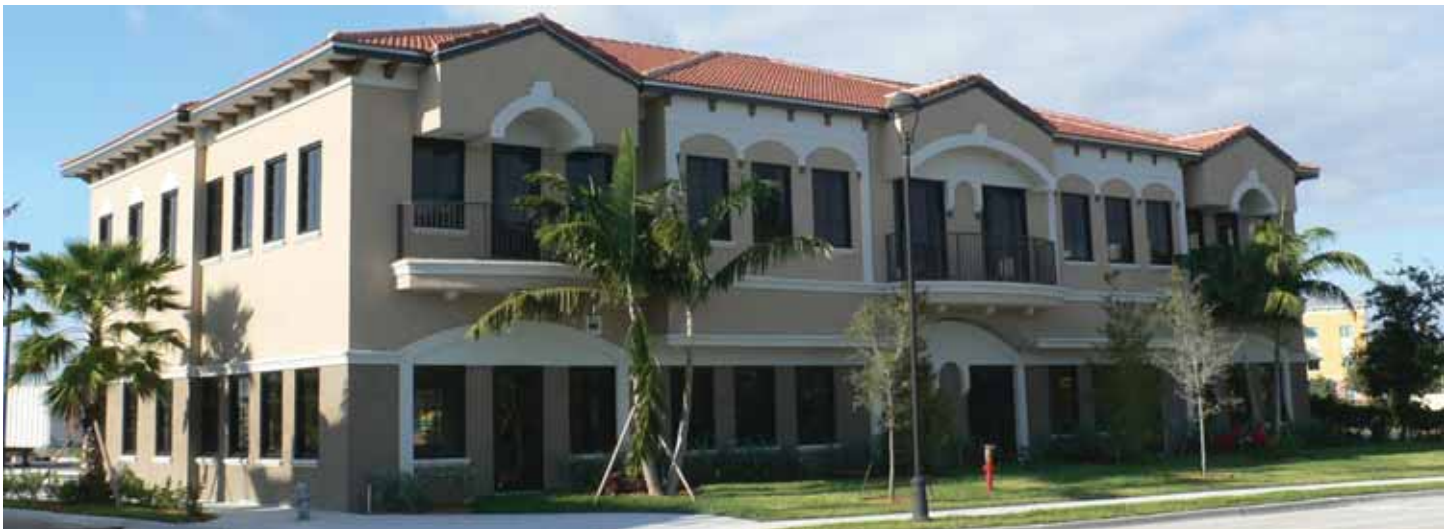
Photo of Beacon Square Professional Campus, Building 9, nearing completion.
